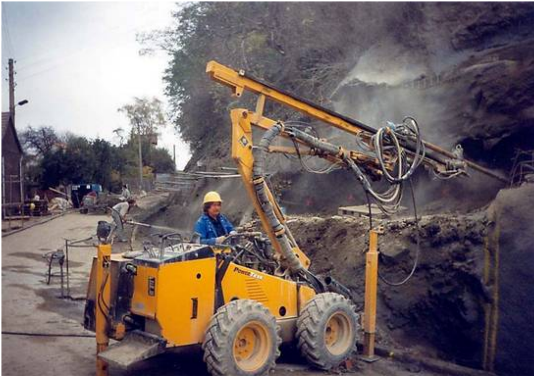
drill rig for slope nailing
