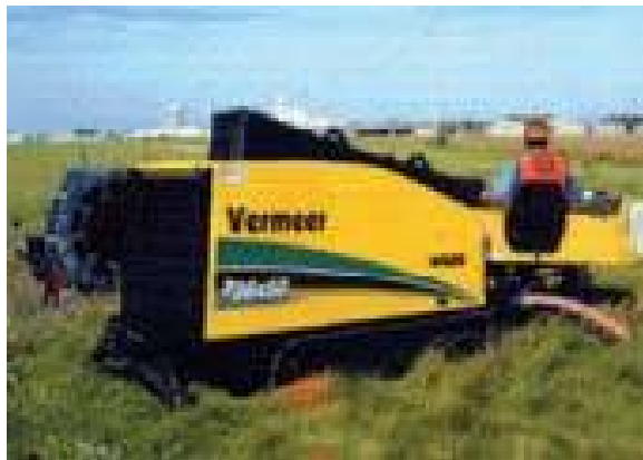
directional rig for controlled drillings
