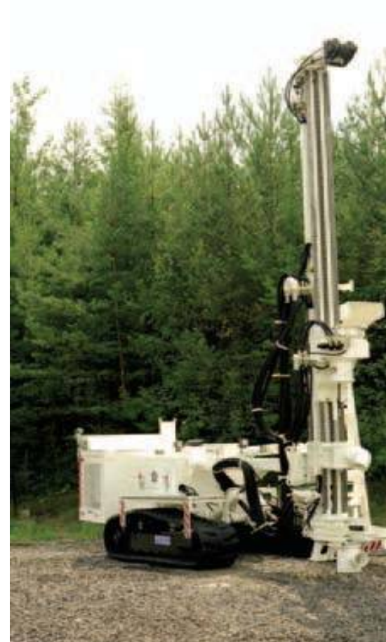
Drill rig for DTH drilling
