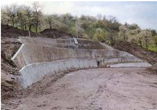
securing a slope
