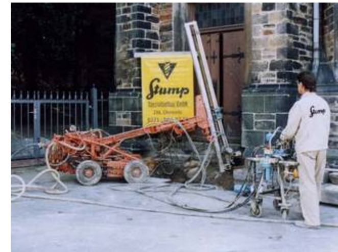
rig at underpinning a foundation
