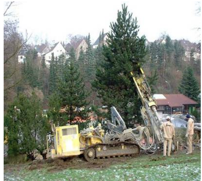
anchor rig at filling cavaties
